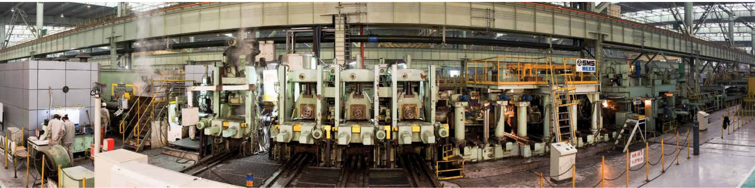
Big River's Osceola, Arkansas Flex Mill™ is the world's only LEED-certified steel mill and is the newest and most technologically advanced flat-rolled mill in North America. The facility is currently in phase two of construction. Photo courtesy of Big River Steel
